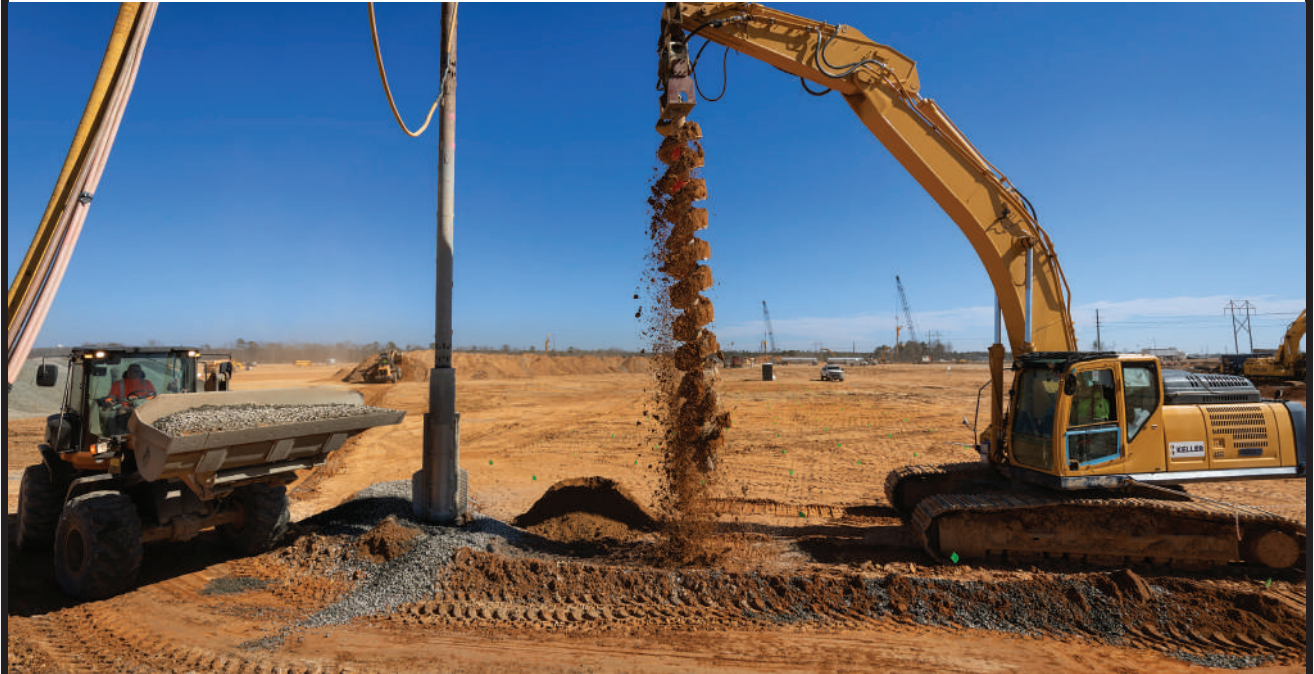
Keller North America ( No. 17 ) is providing ground improvement services over approximately 15 million sq ft of building pads on the $2-billion Scout Motors electric vehicle plant in Blythewood, S.C. The primary scope of work is the installation of aggregate piers with varying depths of 5-30 ft. The facility is scheduled to start production in 2026.
